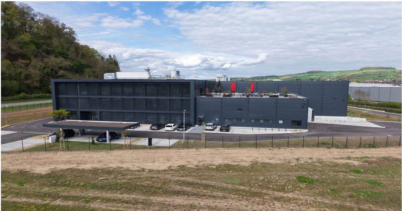
New building, Wutöschingen, 2026 · Roof terrace and PV system
