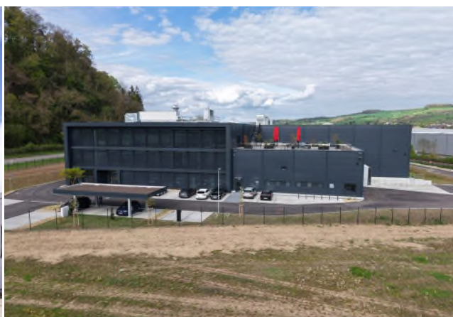
New building, Wutöschingen · Operational from 2026
