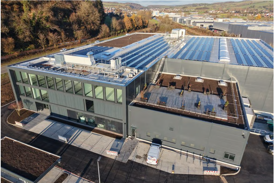
PV system, 460 kWp, on the roof of the new building · Aerial photo, November 2025
